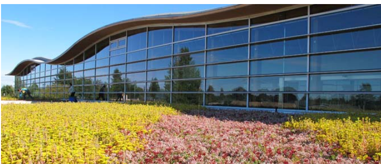
STORM WATER ROOF FILTRATION
